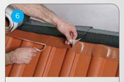
Remove the release paper from the adhesive butyl cover on one side and stretch the fleece slightly at the top to facilitate air flow and stick down. Repeat on other side.
