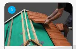
Fix the ridge batten into the **Rapid Ridge Batten Holder** and lay the tiles as normal across the whole roof.
