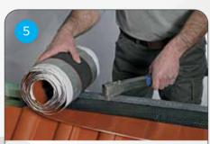
From the gable end roll out the Rapid Ridge Weather Barrier Fleece ensuring there is 75mm cover each side of the top course of tiles and on any overlaps, then secure in place at 300mm centers through the reinforced spine of the fleece with staple gun.
