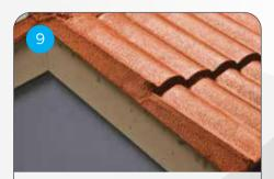
At the gable ends we recommend filling gaps with Flexim roof putty (a ready to use permanently elastic roof mortar). Once completed the finished roof provides a mortar and pointing free ventilated roof.
